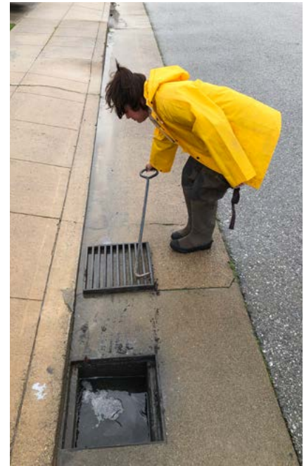
Vector Control Technician Vanessa uses a manhole cover hook to lift a storm drain cover to check for clogs in the pipe.
