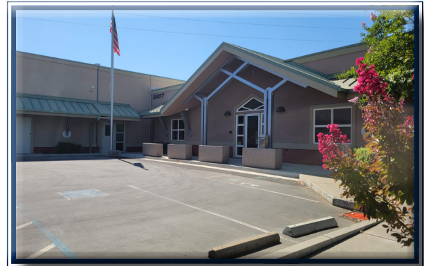
SOUTH PLACER MUD RENOVATED ADMINISTRATION BUILDING
