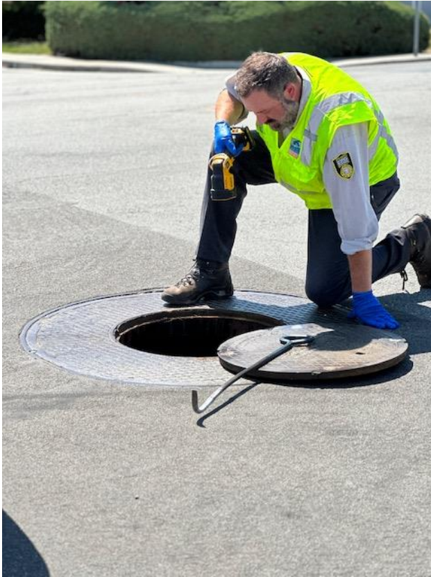
(Left) Vector Control Technician David Allen inspected a storm water vault in San Mateo for mosquitoes.
