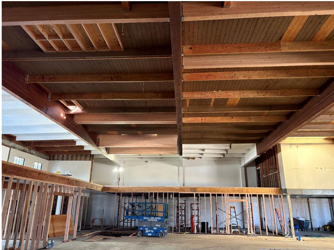
Structural ceiling blocking related to the earthquake retrofit and wall framing for first floor rooms
