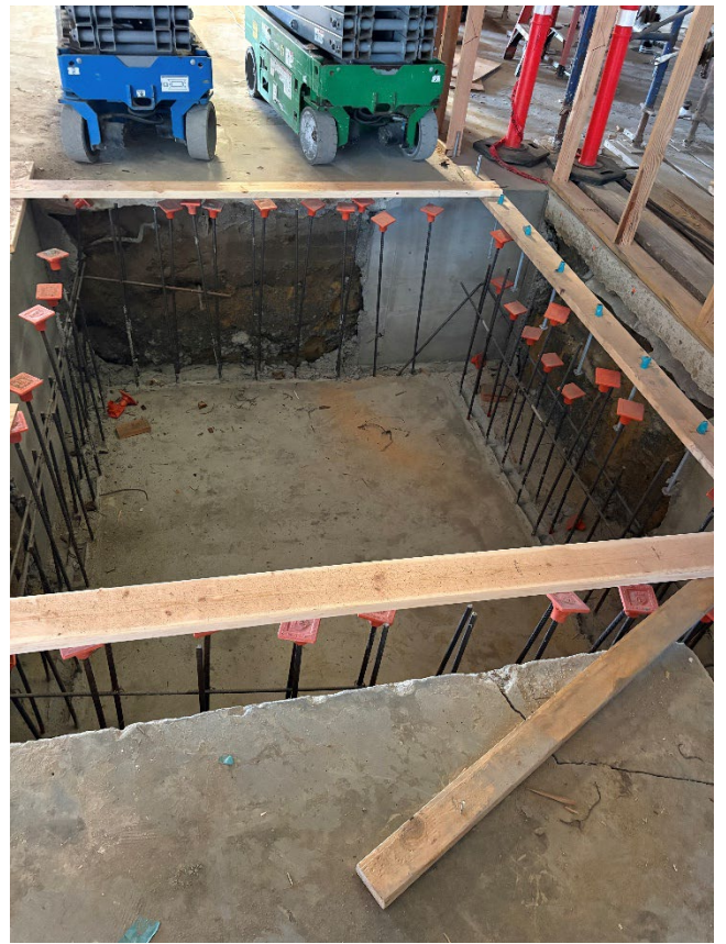
Base of elevator shaft
